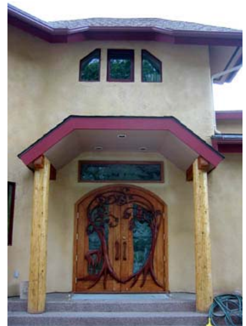
The Waldorf on the Roaring Fork, is the largest straw bale building in Colorado
